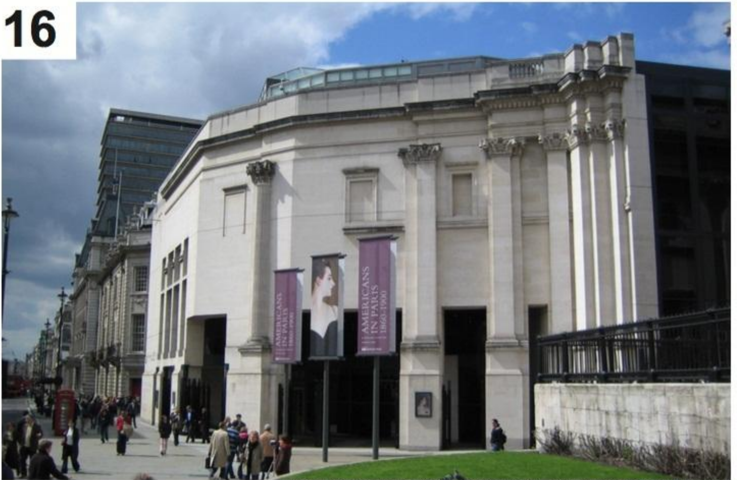
National Gallery extension (Sainsbury Wing), 1982 – 1985, Venturi Scott Brown architects
